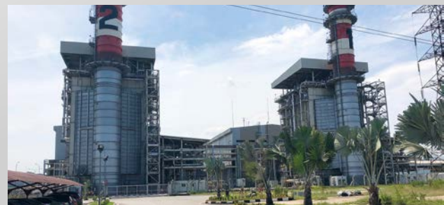
Combined Cycle Power Plant (CCPP) in Southeast Asia
